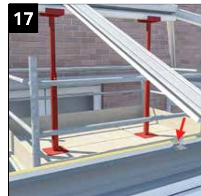
Depending upon the lantern size and options requested, fit hub end transom bar and / or side transom bars. If specified on the job, remove nuts from bolts in transom position and fit transom bar over bolts. Re fit nuts and hand tighten. Check that ridge is level and fully tighten nuts on all bars.
