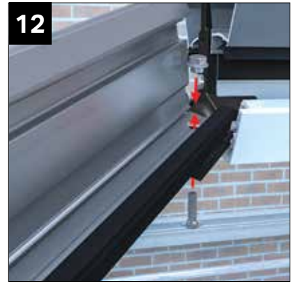
Using NUTS and bolts (SHBC001S - found in BURBOX), locate each hip bar and secure to radius end by hand tightening nuts.
