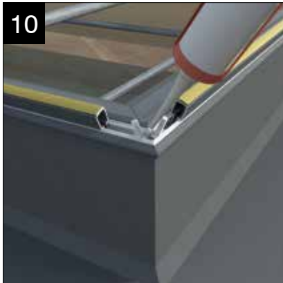
Once rider rail is fitted, seal corner joints.
