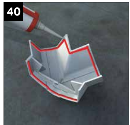
40 Apply generous bead of MS polymer to the underside of the external cover as shown above.
