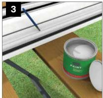
Finally, apply an air drying top coat with a fine brush.
