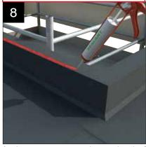
Apply a generous, continuous bead of sealant to the outer perimeter of the top surface of the kerb.
