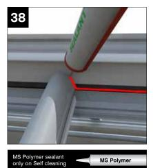
Seal along the ridge baffle where it meets the glazing and over any bar where it meets the ridge.
