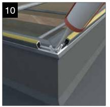
Once rider rail is fitted, seal corner joints.
