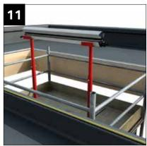
Prop ridge in position using suitable supports, centralising between rider rail. (When the ridge features aluminium painted intenal finish it will need to be protected whilst supporting).
