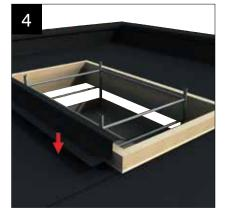
Apply membrane as per manufacturers guidelines. Wrap the membrane up side of the kerb and over the top of the kerb ensuring that a watertight finish is achieved.
