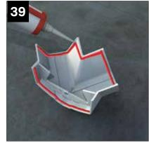
Apply generous bead of MS polymer to the underside of the external cover as shown above.
