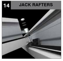
The 2 part jack rafter kit is already fitted to the hip and jack rafter. Ease back the jack rafter undercladding. Each jack rafter kit is supplied with a number of washers. Trial fit the jack rafter and check that the glazing platforms are level. Adjust if necessary by adding or removing washers between the two part connecting kit, then tighten the nut. NOTE: If aluminium internal claddings are being used, fit hip internal cladding prior to fitting jack rafters.
