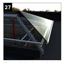
Lift glass units into place onto the glazing bars. When fitting units along the ridge, lift the unit slightly and push into the ridge, then lower onto the rider rail glazing support. Centralise the glazing between the glazing bars. If necessary, pack out on each side.
