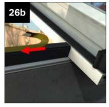
Peel back a small tab of the protective film on the glazing support from the rider rail and the ridge. (ready to be pulled away when the sealed units are finally in position).
