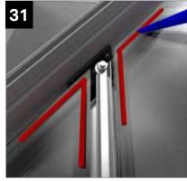
If the lantern has jack rafters. At the corners of the glazing that meet the jack rafter bracket, apply MS polymer to the surface of the glazing as shown above to create a barrier. This should be positioned towards the edge of the glazing as to be obscured by the top caps once they are installed.
